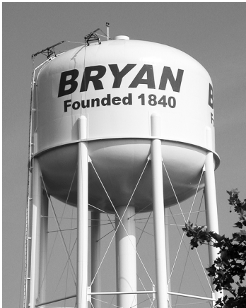
Final phase of fresh paint on the 400,000 gallon tower
