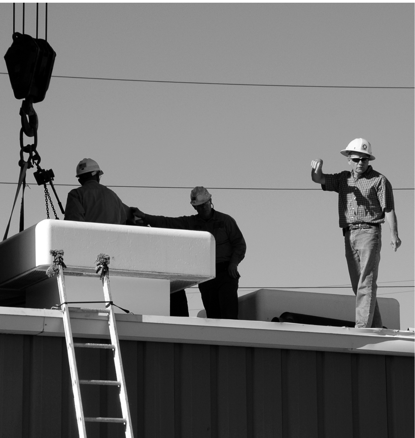
Power Production Superintendent Matt Killion directs the crane operator lowering the rebuilt starting diesel engine through the roof of the building that houses the Westinghouse gas turbine generator.
