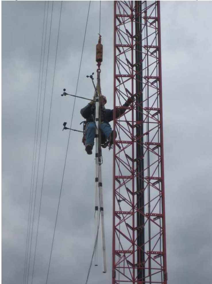
Figure 1: Boom Installation on Communications Tower at Bryan
